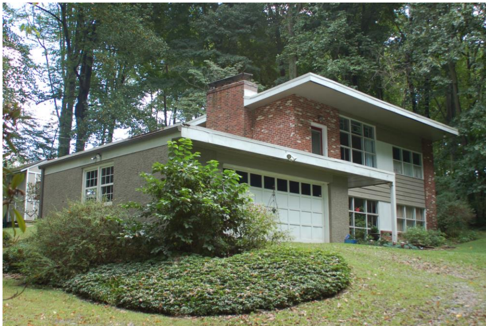
North and West (front) Elevations, House
