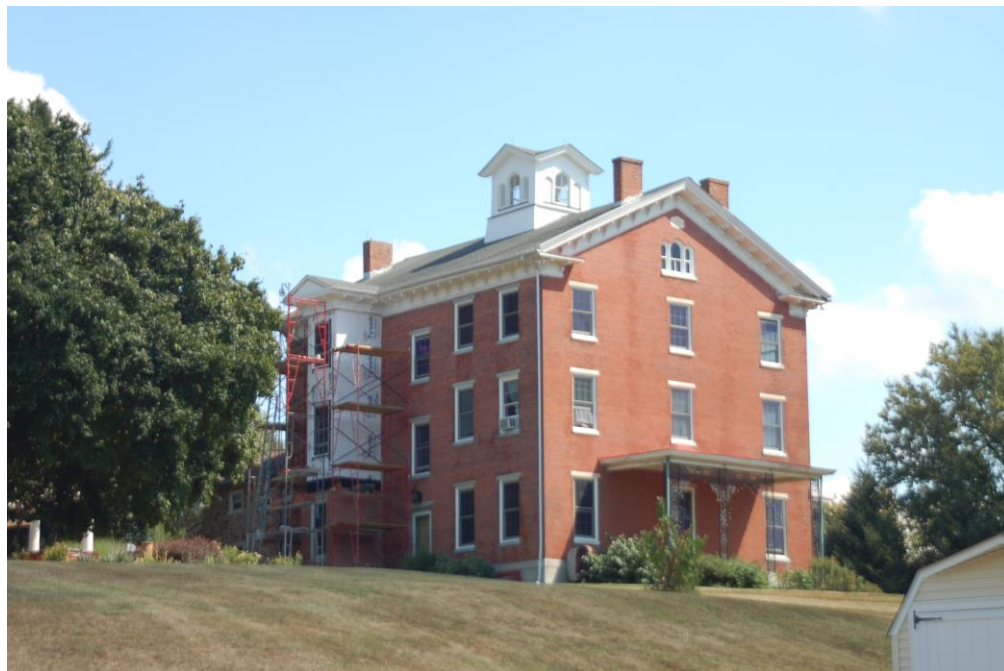
North (back) and West Elevations, John Woodward [II] Addition, Thomas Woodward House in Center Background
