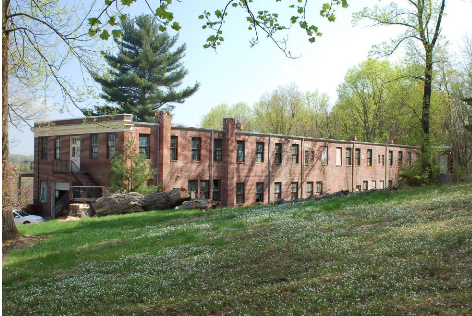
West and South (back) Elevations, St. Vincent dePaul School
