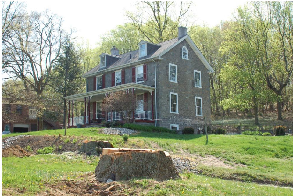
North (front) and West Elevations, House, with St. Vincent DePaul School in Left Background
