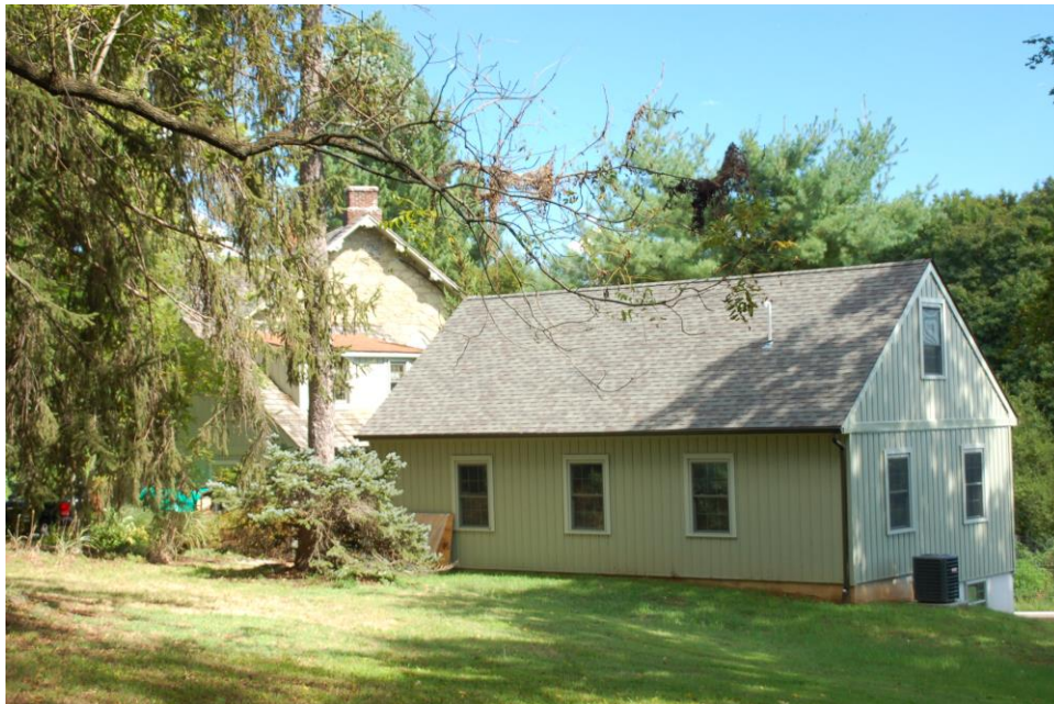
North and West Elevations, New Outbuilding with House and Garage in Background
