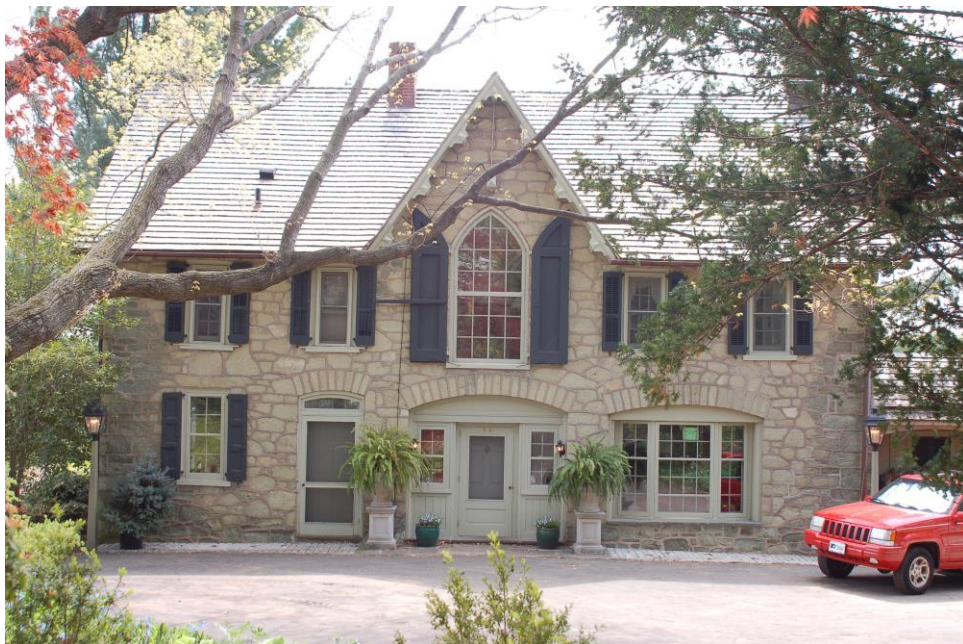
North Elevation, House
