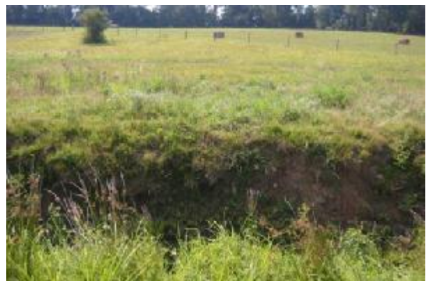
Existing stream bank erosion.
